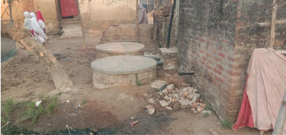
**Figure 5: Inappropriate design of the twin pits, where the distance between two pits is less than 1 m.**
