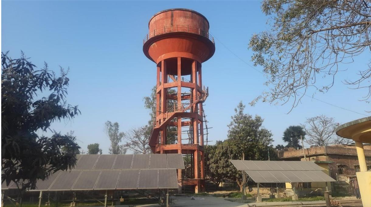
**Figure 13: Overhead Tank for Piped Drinking Water Supply System in Rajpur Municipality.**
