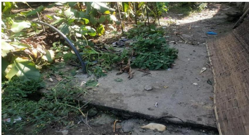
**Figure 6: Lined Tank with Impermeable Walls and Open Bottom in household of Phungling Municipality.**
