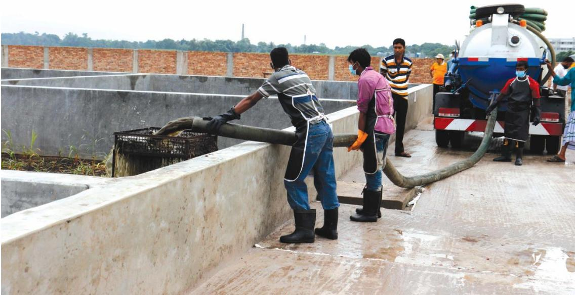
**Figure 5: Sludge dumping from vacutags at planted drying bed (Photo courtesy: Practical Action, Bangladesh).**
