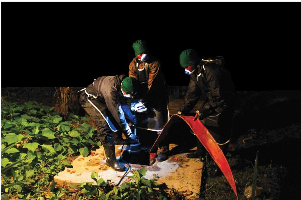
**Figure 6: Desludging of septic tank with submersible pump (Photo courtesy: Practical Action, Bangladesh).**
