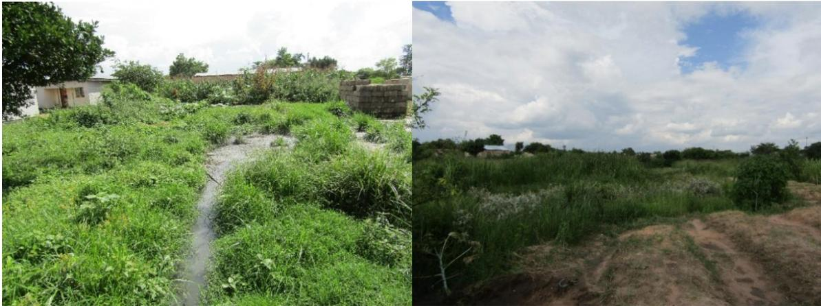
**Figure 5: Blockages in some sections of the sewerage networks for Mansa Town (LHS: A blocked septic tank upstream of the Sparks Wastewater Stabilisation Ponds (WWSPs); RHS: Dry Maturation Ponds indicative of low flows) (Source: Author).**
