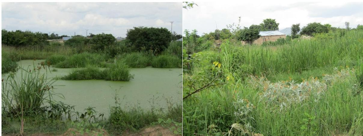
**Figure 7: The Spark WWSPs (LHS: The weed infested facultative pond with sewage in it; RHS: Dry maturation pond infested with weeds) (Source: Author).**
