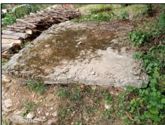
Lined tank with impermeable wall and open bottom.
