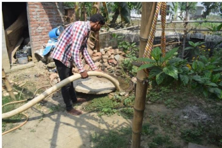
**Figure 9: Private desludger performing emptying of containment.**
