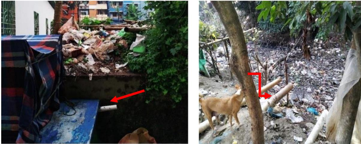
Figure 6: Containment technologies and their connections in Narayanganj. Left: Septic tank connected to the nearby water body. Right: Toilet pipe connected to open drain (Source: Feasibility study 2020-21, DPHE).
