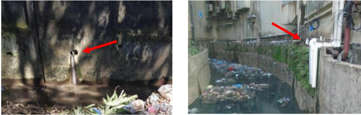
**Figure 6: Containment technologies and their connections in Sylhet. Left: Septic tank connected to the nearby water body. Right: Toilet pipe connected to open drain (Source: Feasibility study 2020-21/DPHE).**
