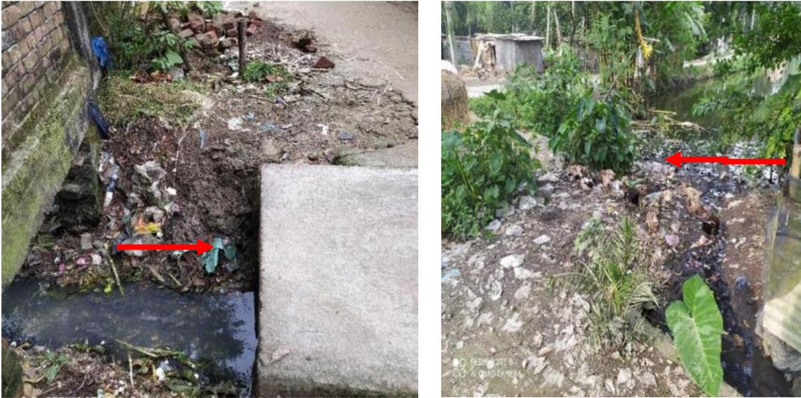
**Figure 6: Containment technologies and their connections in Naogaon. Left: Septic tank connected to the nearby water body. Right: Toilet pipe connected to open drain. (Source: Feasibility study 2020-21/DPHE).**
