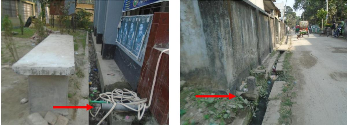
**Figure 6: Containment technologies and their connections in Nilphamari. Left: Septic tank connected to the nearby water body. Right: Toilet pipe connected to open drain. (Source: Feasibility study 2020-21/DPHE).**
