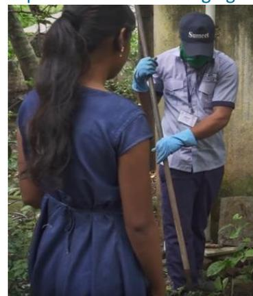
sludge. If the remaining sludge is more than 25mm, excess sludge must be sucked out. 25mm thickness of sludge is retained in the septic tank for allowing micro-organism to be present inside the tank to act on the new incoming faecal waste.
