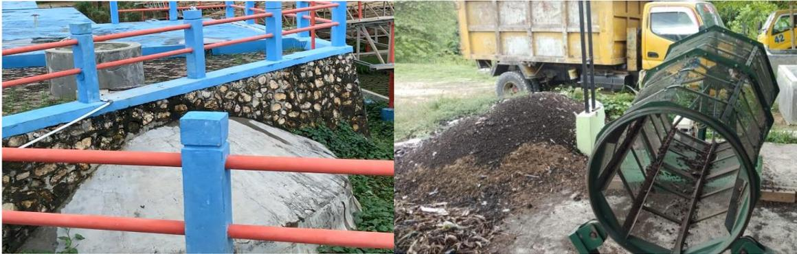
*The biogas digester in the IPLT Gempong Jawa (Banda Aceh) generates gas that can be used as a source of energy (left picture) and the sieving facility used at the IPLT Koya Koso (Jayapura) produces finer sludge particles to be used as a soil enrichment material (right picture).*
