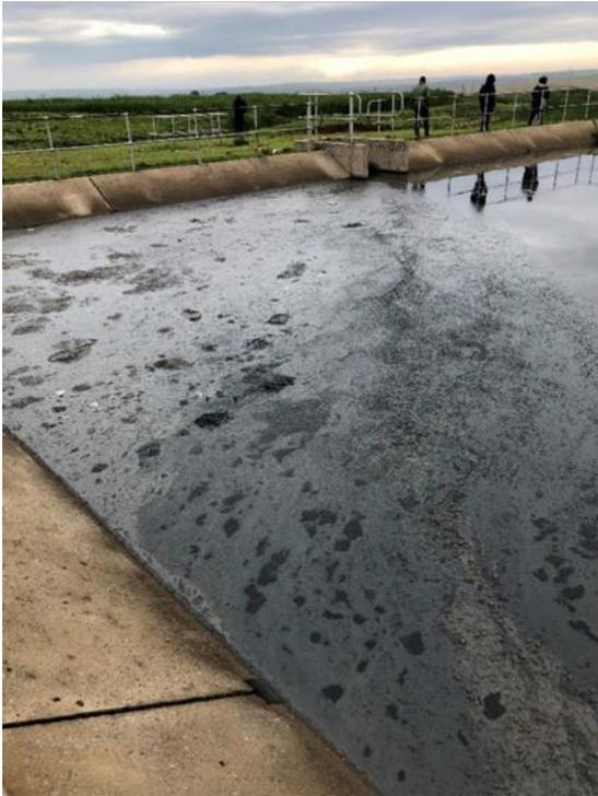
Figure 10: Pond showing accumulated sludge at Dannhauser WWTW (Tweediedale Ponds)
