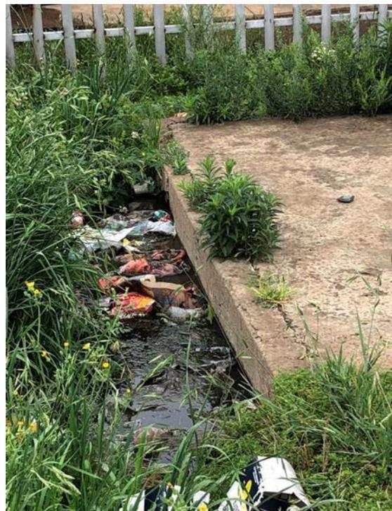
Figure 11: Evidence of wastewater leaking from taxi rank public toilet conservancy tank (Dannhauser)
