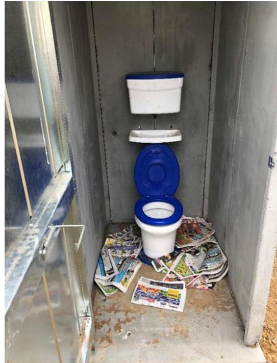
Figure 8: Newly constructed VIP and indicating ability to be connected to water supply (in future, if required)
