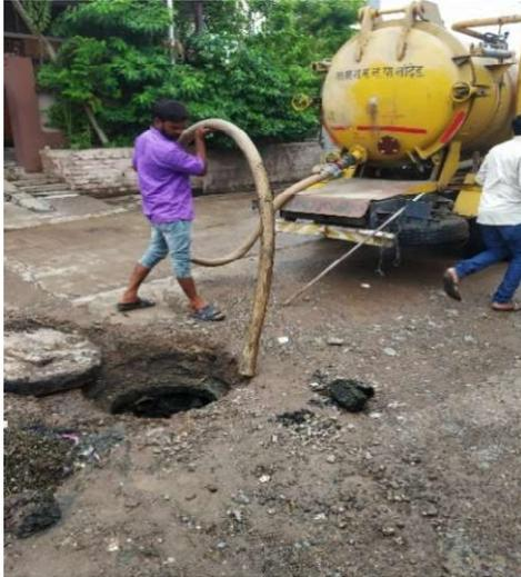
Figure 4: Manual cleaning of blocked sewers in Maganpura of Ward 9 (Abhijit/CSE/2021).
