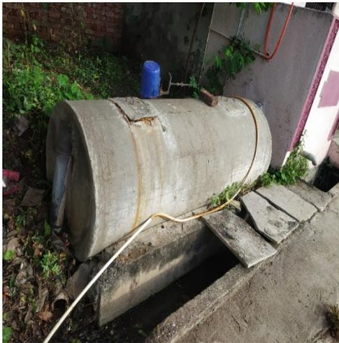
Figure 7: Circular septic tank connected to open drain in Ward No. 01. (Abhijit/CSE/2021).
