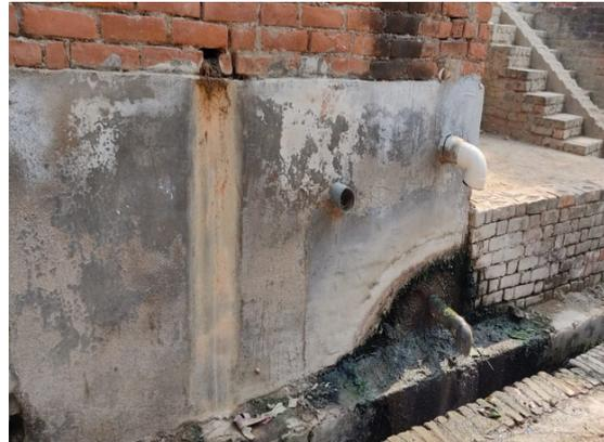
Figure 4: Toilet discharging into open drain.
