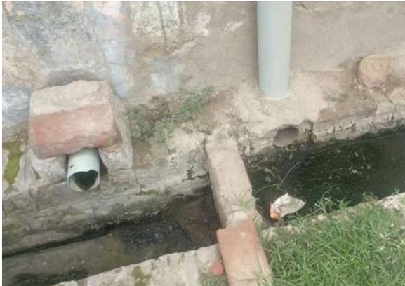
Figure 3: FLT discharging into open drain.
