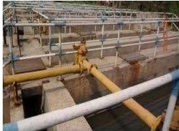
Figure 7: UASB Reactor System at Sajri STP.
