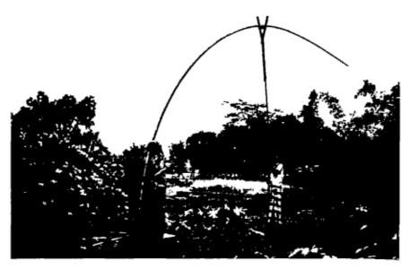
A conveniently located tree provides the ideal form of support during installation and removal of the pump rod, but a bamboo pole can also do the job.
