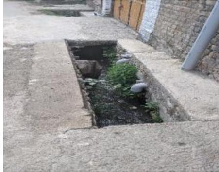
Figure 2: Wastewater is discharged directly to open drains.
