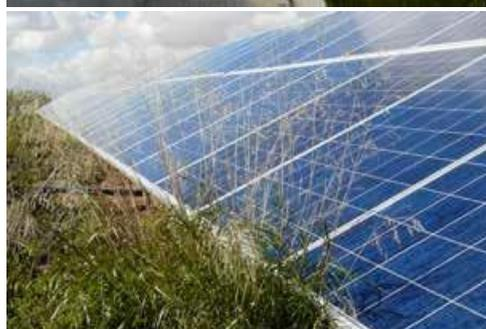
Example of a dangerous cable connection; Galvanic corrosion of a manual tracking system; Limited heat dissipation capability of corroded controller housing; Examples of inadequate maintenance Accumulated grime at the lower end of a PV panel; Example of PV shadowing by not maintained ground vegetation- (Source: Andreas Hahn, 2015)
