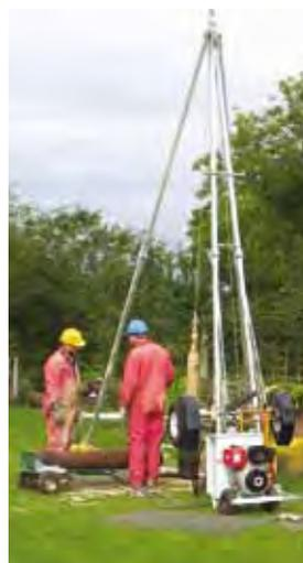
**Figure 4. The Forager 55 cable-trailer rig in use**
