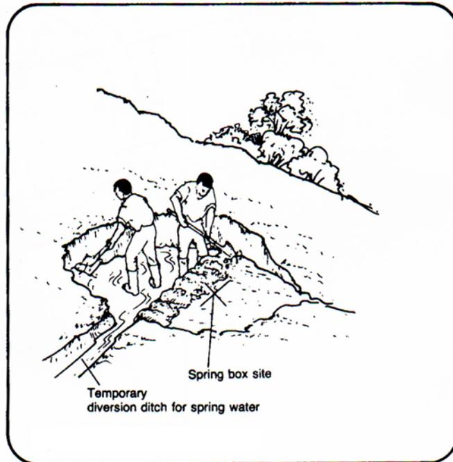
Figure 7: Excavating the spring site. Note temporary diversion ditch
