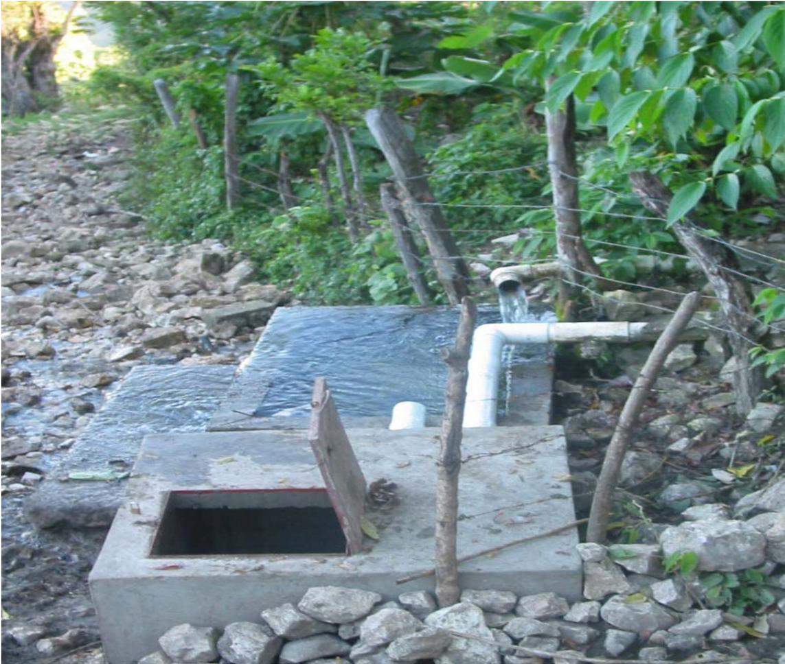
A newly completed spring box in the Dominican Republic. Note old spring box behind the new structure with open top to allow livestock a drink of water. Photo courtesy of Matt Niskanen, 2003.
