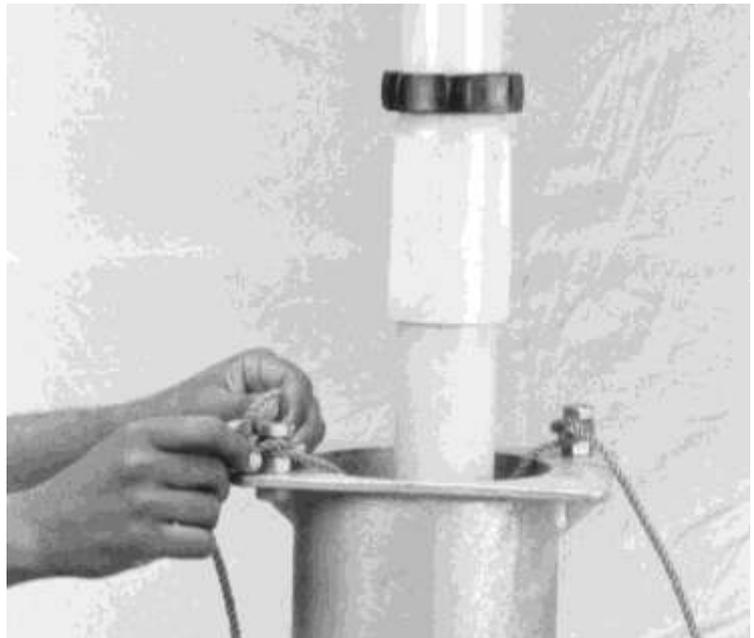
6.1.11 As soon as the last pipe is lowered, the steel cone is inserted and laid to the top flange of the pump stand.
