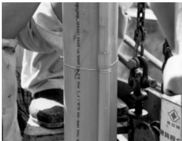
Figure 7.17 Use of small diameter pipe as centralisers
