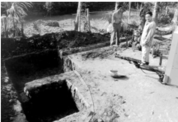
**Figure 2.5** Well proportioned mud pits ready for filling
