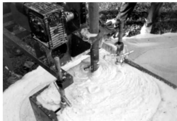
Figure 4.1 *Drilling with stable foam*
