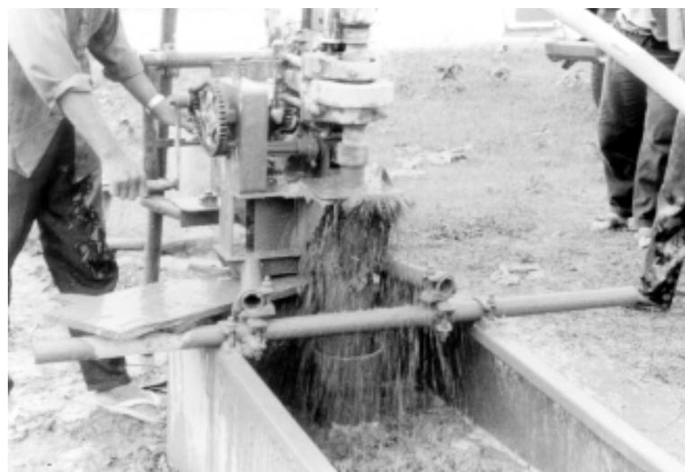
**Figure 3.2** *Drilling with compressed air – having "struck" water*
