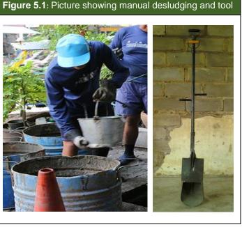
systems. There are also shovels for lower viscosity sludge which a longer lever, additional holders, and a closable reservoir, increasing the operation depth and the emptying rate. The manual emptying is used in inaccessible regions where the willingness to pay for de-sludging is low.
