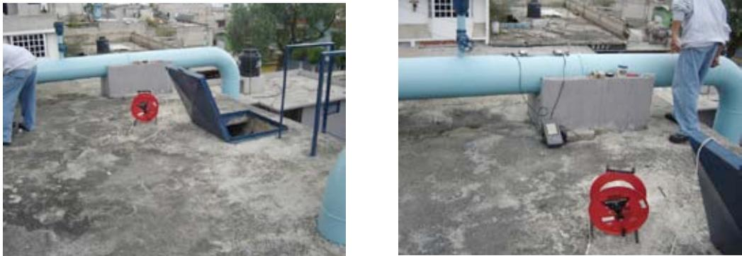
If the level changes position significantly while measuring in a suction pit or water tank, it is important to take simultaneous measurements of flow, pressure, and electrical parameters. The value can be negative or positive, depending on whether the level is below or above the reference level.
