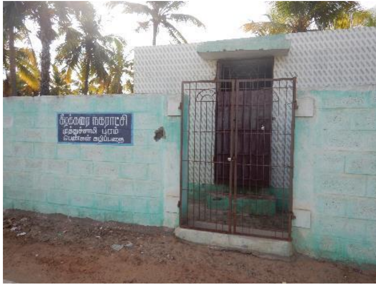
Figure 3.7: Public toilet in Muthuswamipuram, Kilakarai
