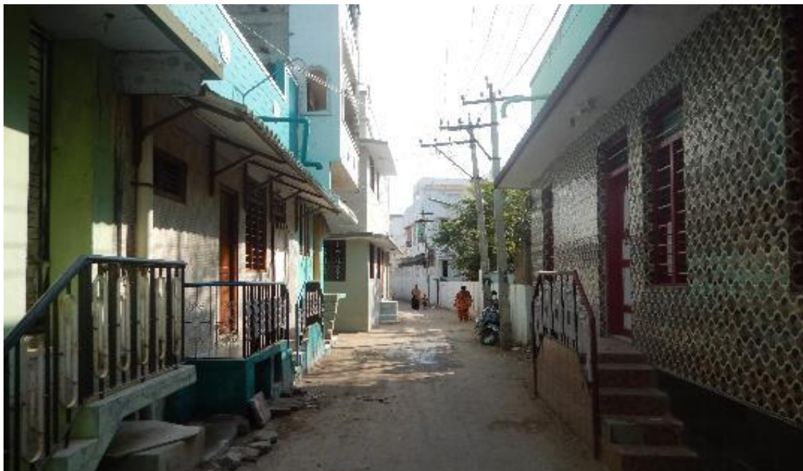
Figure 3.17: Absence of storm water drains
