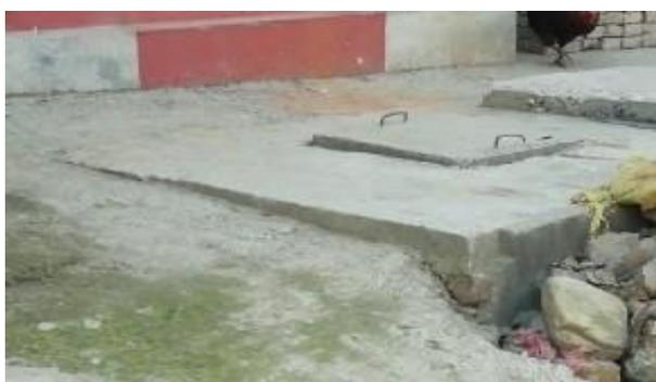
Figure 2: Containment system with manhole cover (HHs survey, 2019)
