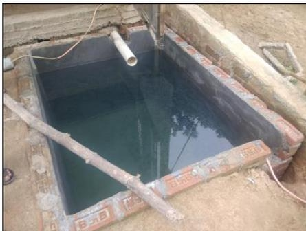
Figure 3 : under construction single chamber fully lined tank
