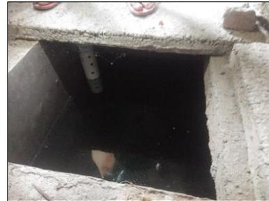
Figure 2 : Septic tank connected to open drain
