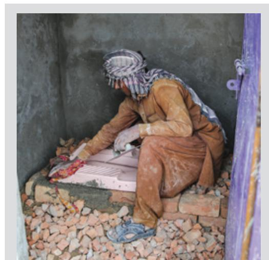
WC fixed into substructure
