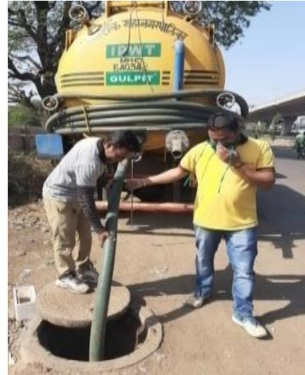
**Figure 4: Discharge by vacuum truck in trunk sewer (Source: Ekta/CSE, 2020)**
