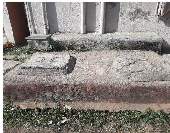
**Figure 3: Two chambered ST in a HH (Ward no. 4) (EKta/CSE, 2020)**
