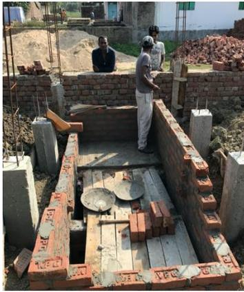
**Figure 2: Septic tank with three chambers under construction**
