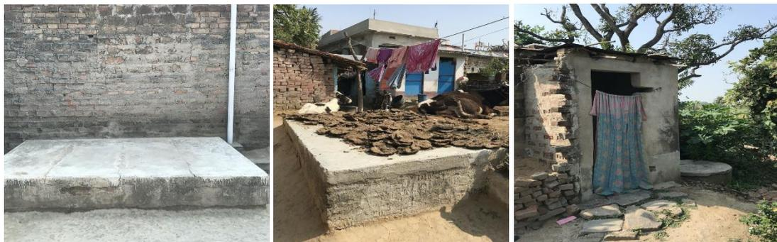
**Figure 1: Septic Tank equipped with ventilation pipe, Fully Lined tank and Lined Pit semi-permeable wall and open bottom (Source: Harsh/CSE, 2020)**
