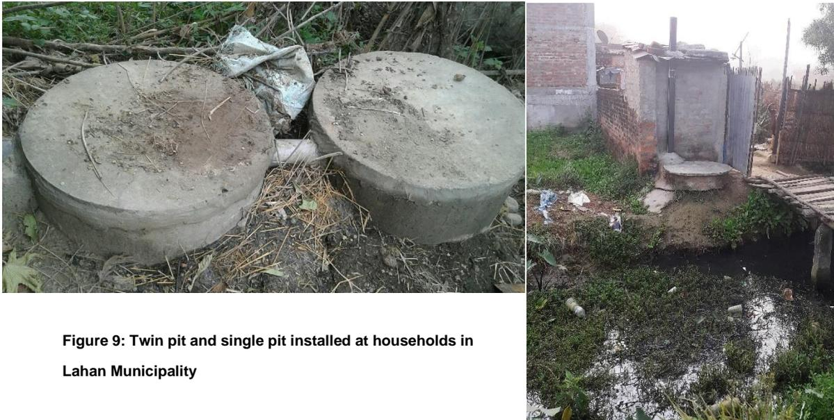
**Figure 9: Twin pit and single pit installed at households in Lahan Municipality**
