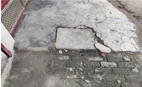
**Figure 2: ST with 2 chambers found in Shiv Colony, half of which is inside the house and half is outside for emptying (Abhishek/CSE, 2020)**
