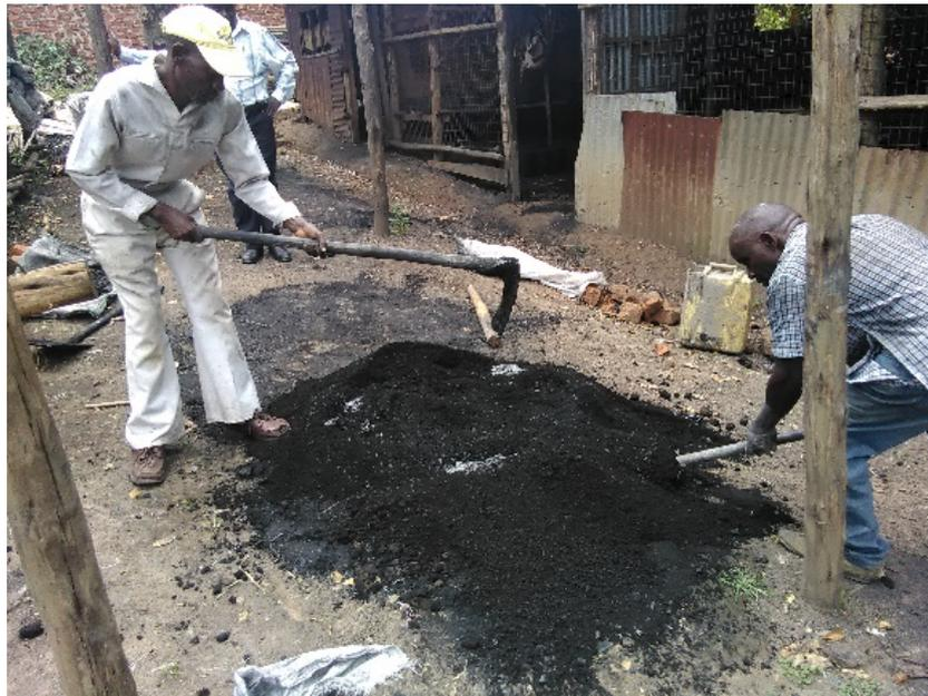
Figure 12: SEACO team being trained in FS inclusion as a briquette input. [Photo credit: Water for People - Uganda]
