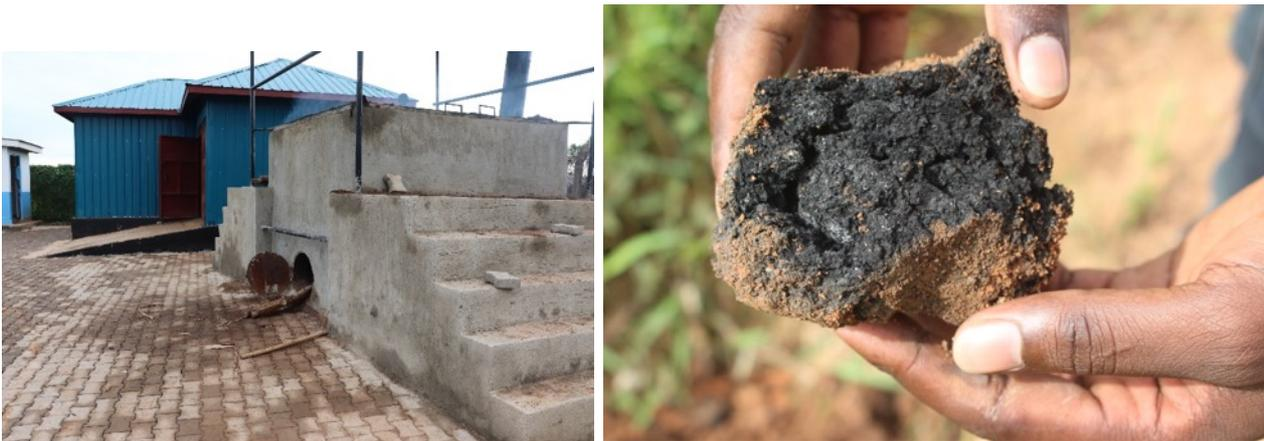
Figure 20: Carbonisation unit at Lubigi NWSC and carbonised sludge on the right.
