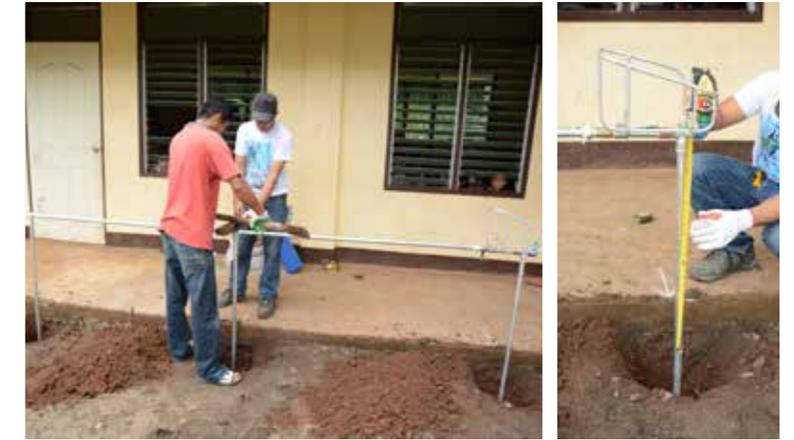
Using a water level, make sure that the water pipe is horizontal and the posts are upright.
