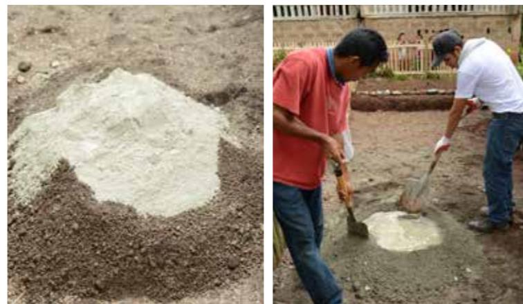
Pour equal part of wet sand-cement mix in the three holes.
