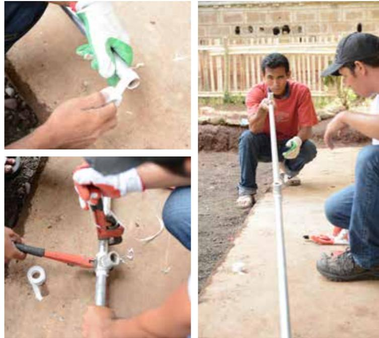
Connect the bucket component to the water pipe in the provided union patente. Don't forget to apply Teflon on the patente before fastening,
