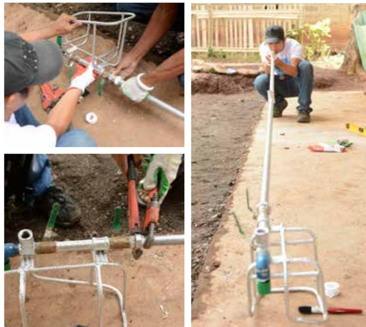
Attach the three posts to the free end of the welded tee connections. No Teflon is necessary since water will not flow in this side.
