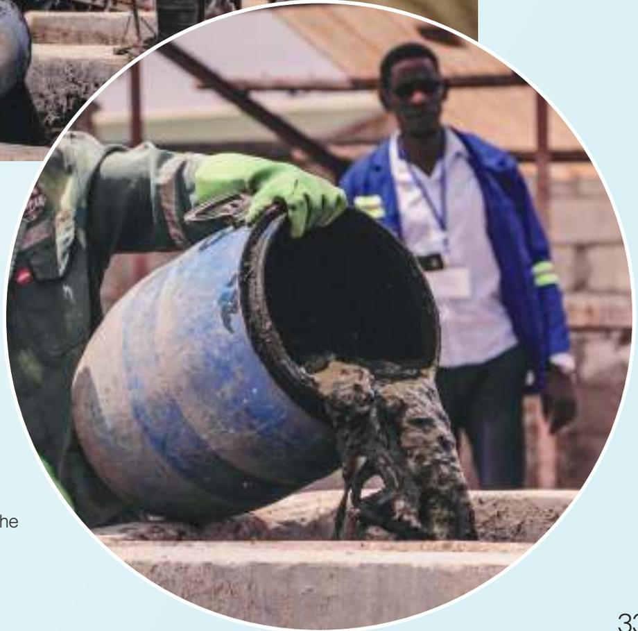
The sludge is poured into a feeding bay where solid matter is fished out using equipment. Screens on the side walls of the feeding bay help trap the solid waste.
