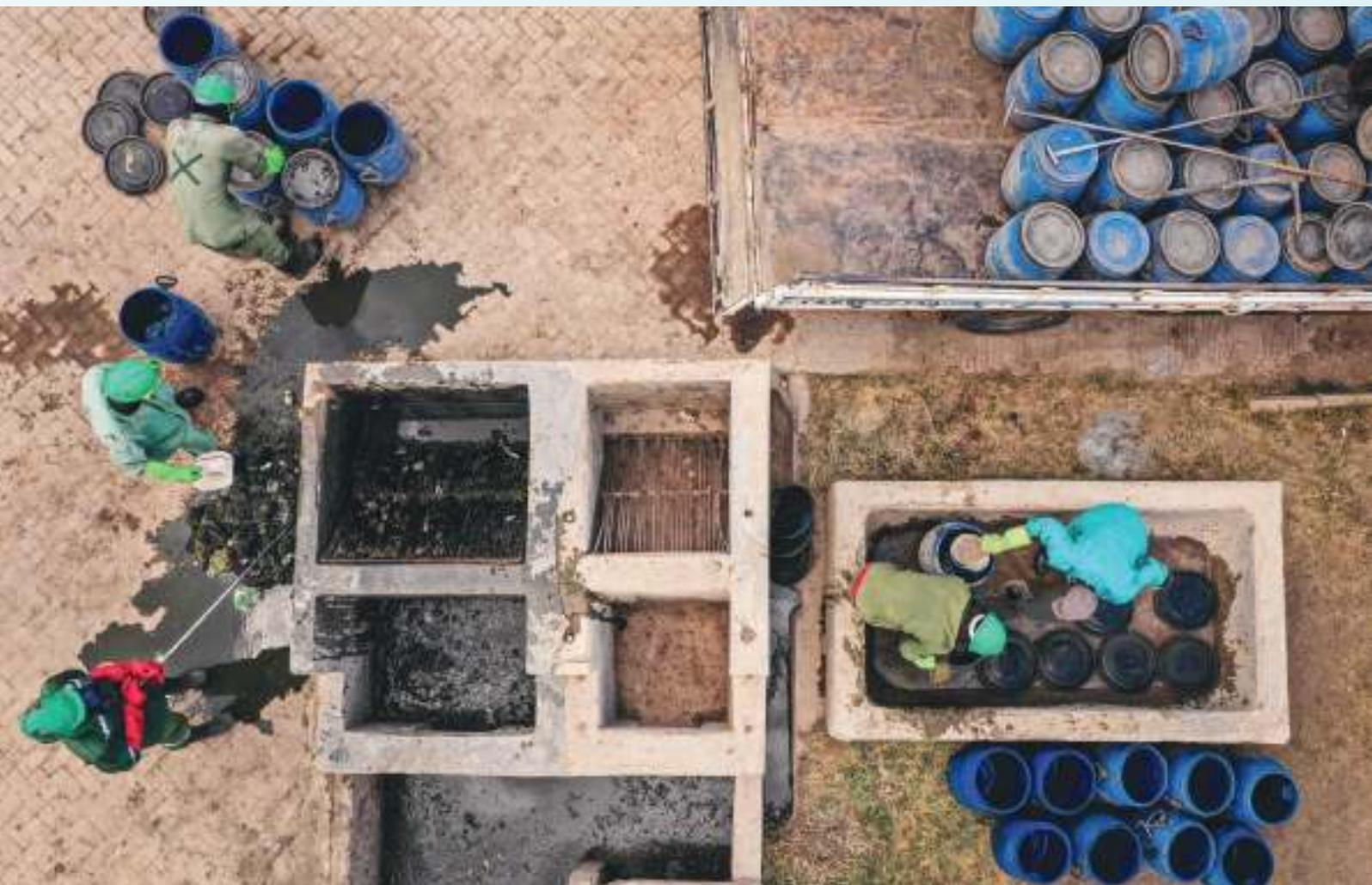
The solid matter that is raked out is washed thoroughly, dried on metal racks and later sent to the landfill nearby. Washing the solid waste removes the faecal matter, facilitating faster drying.
