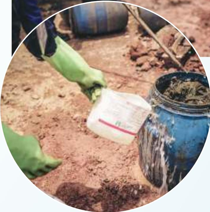
One by one, the other emptiers take their turn using the scoop to remove sludge and fill the barrels. Once the barrels are filled, one half of the team starts disinfecting the barrels and loading them on to the trucks while the others close the opening and clear the area.
