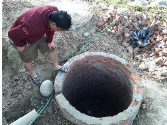
Figure 8 : A soak pit constructed to discharge effluents.
