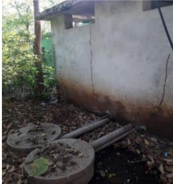
Figure 9: Toilet connected to lined pits.
