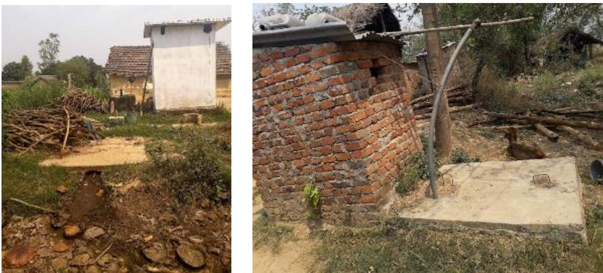
Figure 8: Toilet connected to biogas digester and a fully lined tank.
