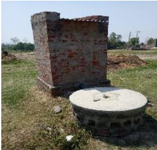
Figure 4: A concrete ring pit
