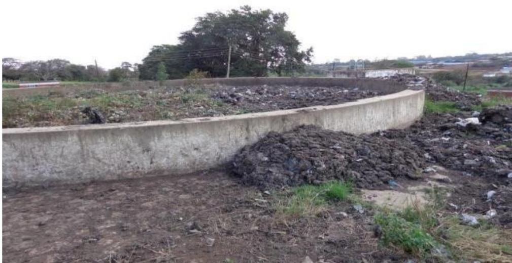
**Figure 12. Drying beds at Soche WWTP (Source: Yesaya, 2016)**
