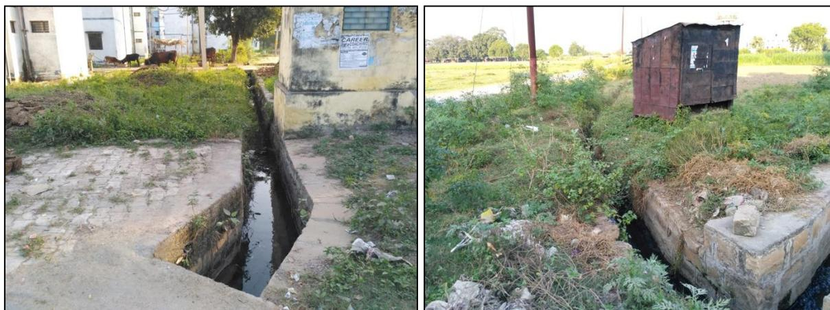
Figure 3: Wastewater conveyed through open storm-water drains (Source: Bhavik/CSE, 2016)
