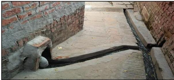
**Figure 1: Septic tank connected to open drain (source: Bhavik/CSE, 2016)**
