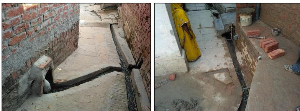
Figure 2: Septic tank with effluent pipe connected to open drain (Source: Shantanu/CSE, 2016)
