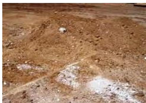
Figure 14 Lime stabilization
