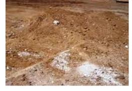
Figure 14 Lime stabilization
