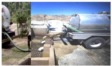
Figure 13 Sludge disposal into inlet chamber of STP
