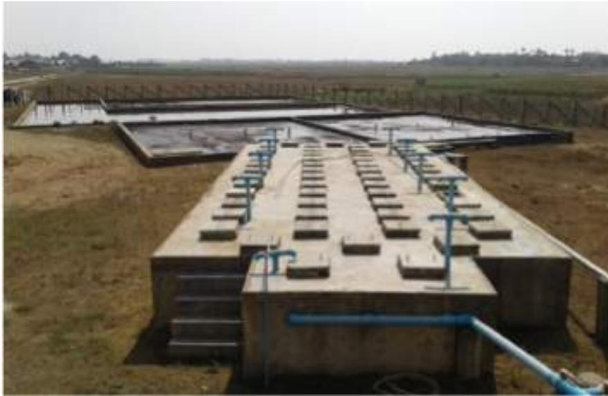
Figure 10. Settler and Aerobic Baffle Reactor within STS Sittwe (Pageud, 2017)
