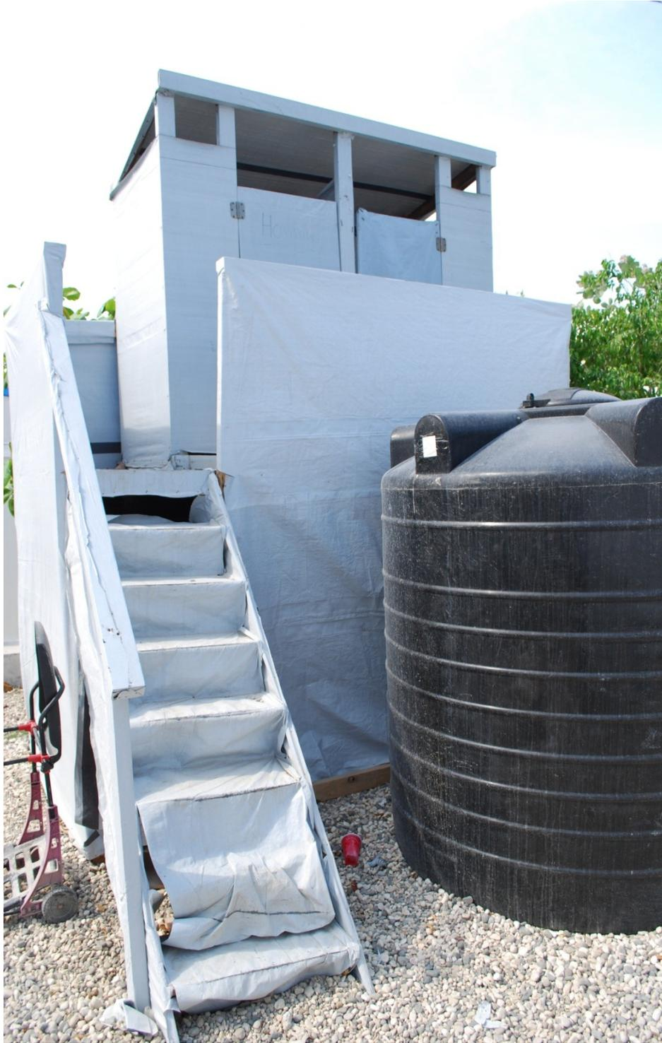
*Figure 3: Storage of latrine wastewater in a 2.4 m<sup>3</sup> 'Tuff Tank'*
