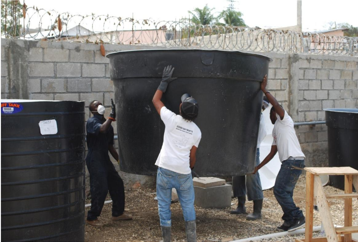
*Figure 1: Installation of an empty 3.8 m<sup>3</sup> 'Tuff Tank'*
