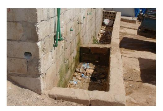
Tanks with taps can facilitate handwashing for more than one person at a time and may be locally constructed from sourced materials.
