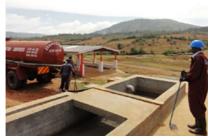
Decentralised Treatment Facility in Machakos
