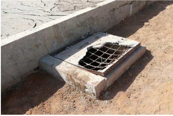
Figure 4: Damaged cover, Cambérène FSTP
