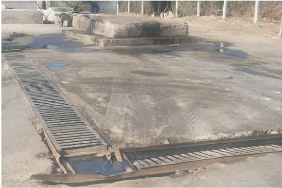
Figure 5: Damaged drain, Rufisque FSTP
