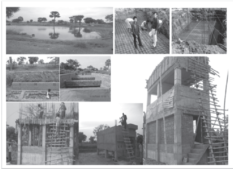
Construction of Surface Water Scheme
