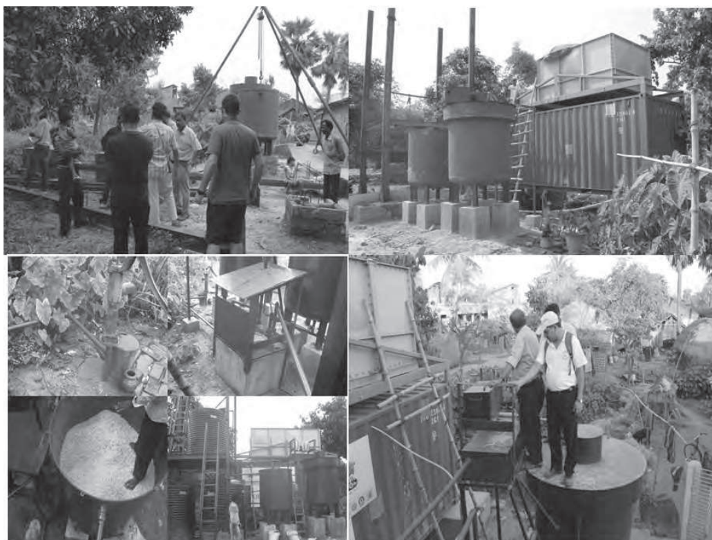
Construction of Groundwater Scheme
