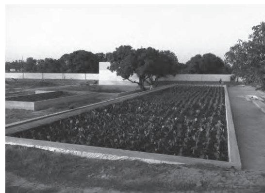
HORIZONTAL FLOW CONSTRUCTED WETLANDS
