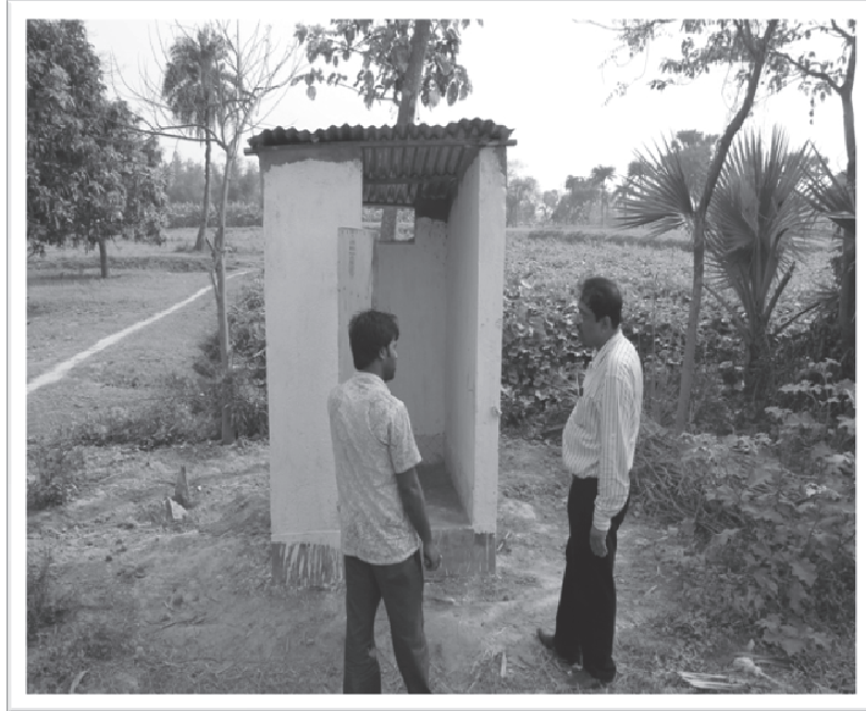
Constructed Sanitation Unit
