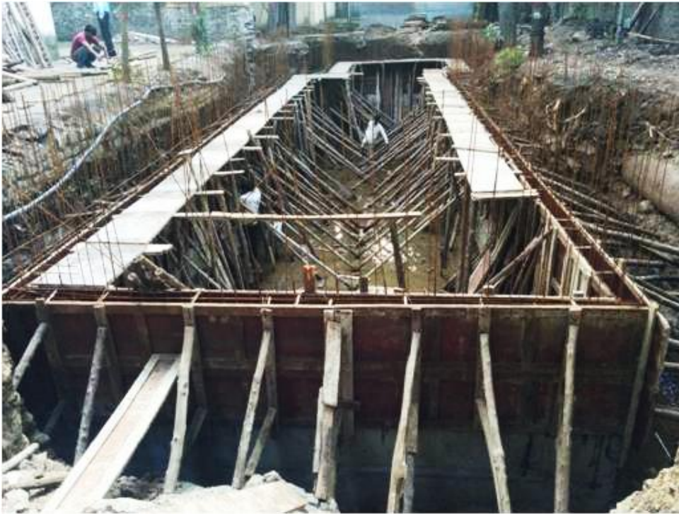
DTS 100 (under construction)
