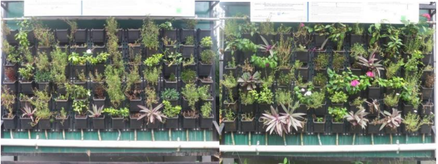
Vertical garden for treating greywater from an office building
