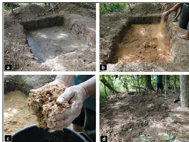
**Fig. 5:** Ditch previously excavated to receive sludge that results from tank maintenance. A) ditch with sludge. B) sawdust being added. C) sawdust. D) ditch covered with soil.
