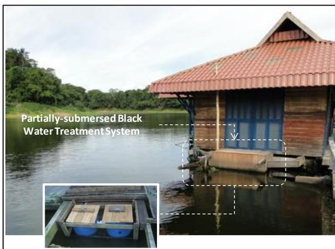
**Fig. 3:** Floating home with a partially-submersed black water treatment system.
